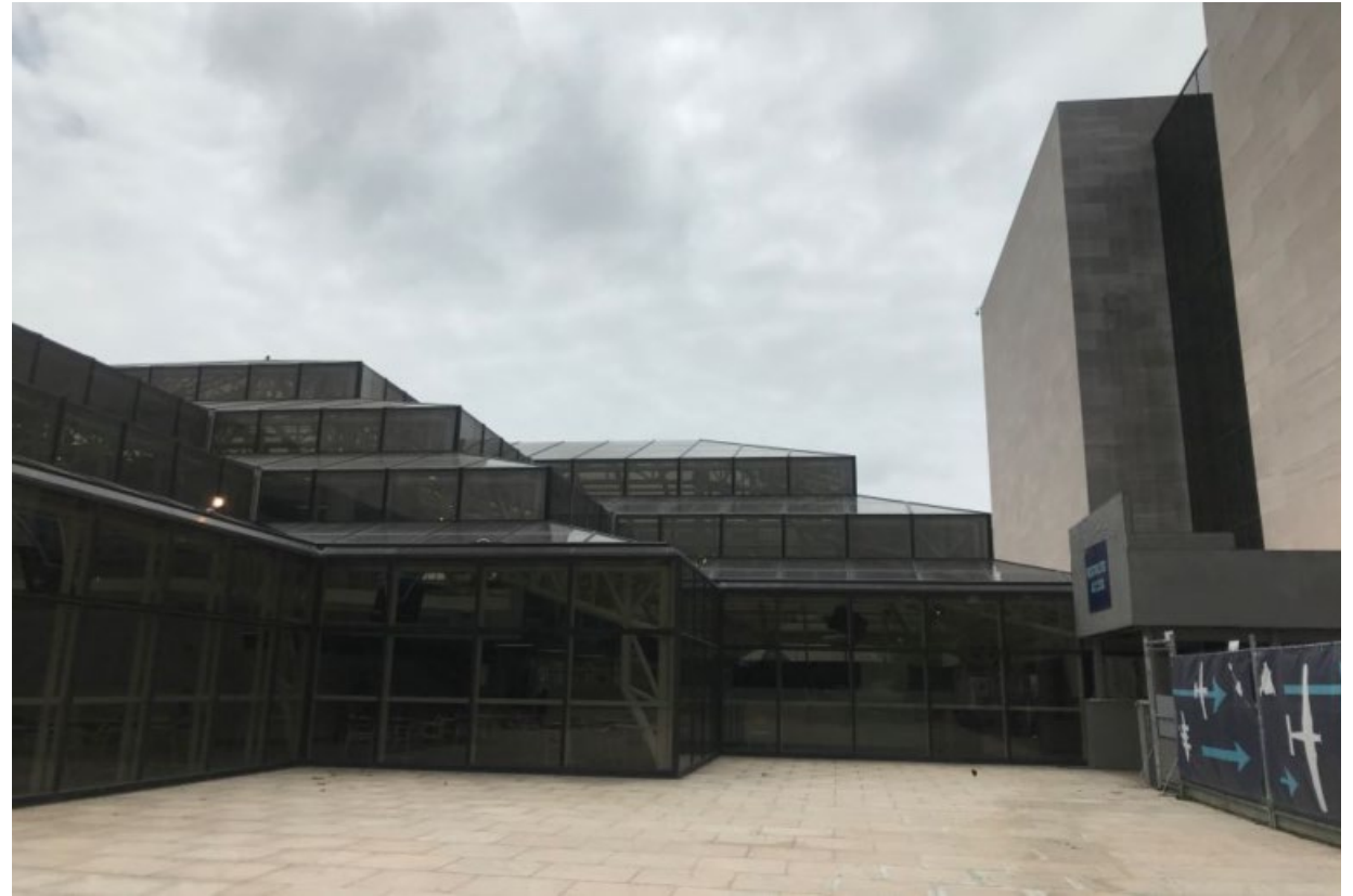
Northwest Corner of the Restaurant Addition, 2020.
