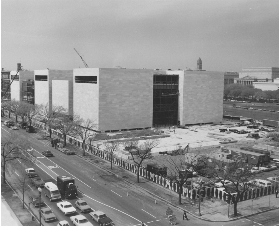
NASM and East Terrace Under Construction, c. 1974.
