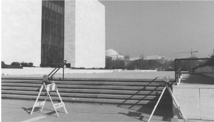
East Terrace, Looking North, c. 1976.
