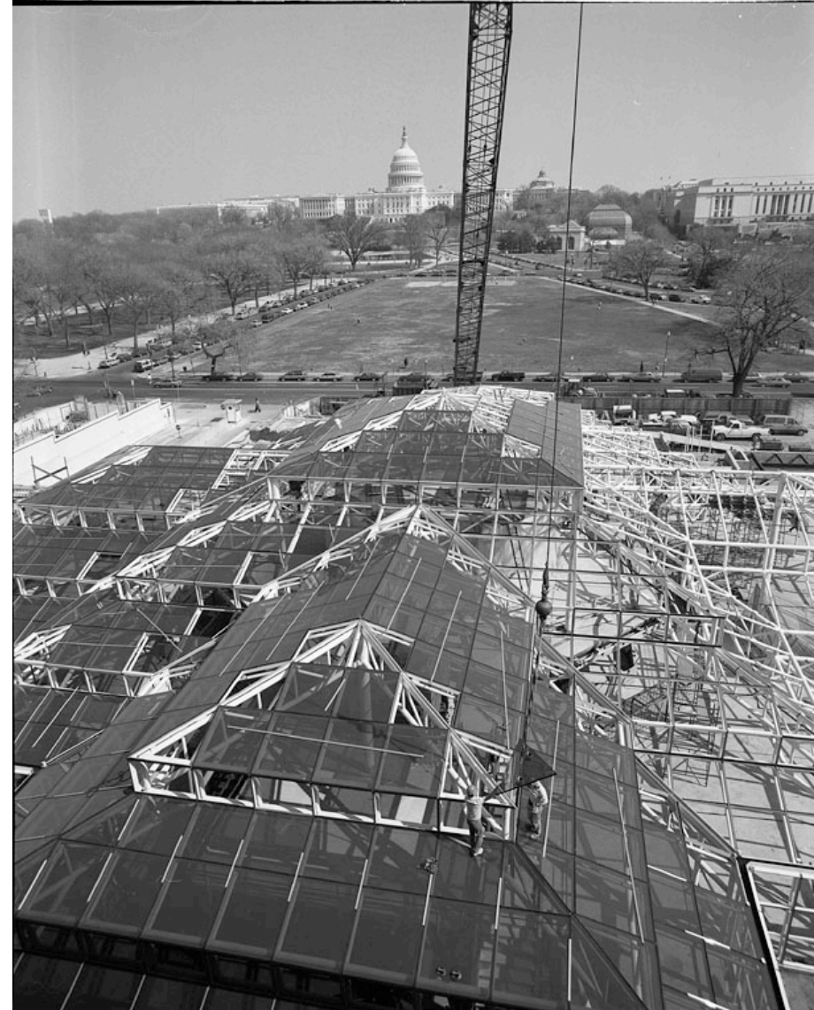
Restaurant Addition Under Construction, c. 1988.
